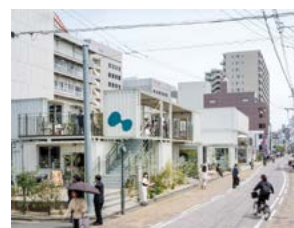
HAROW広島道外観 ©YASHIRO PHOTO OFFICE
